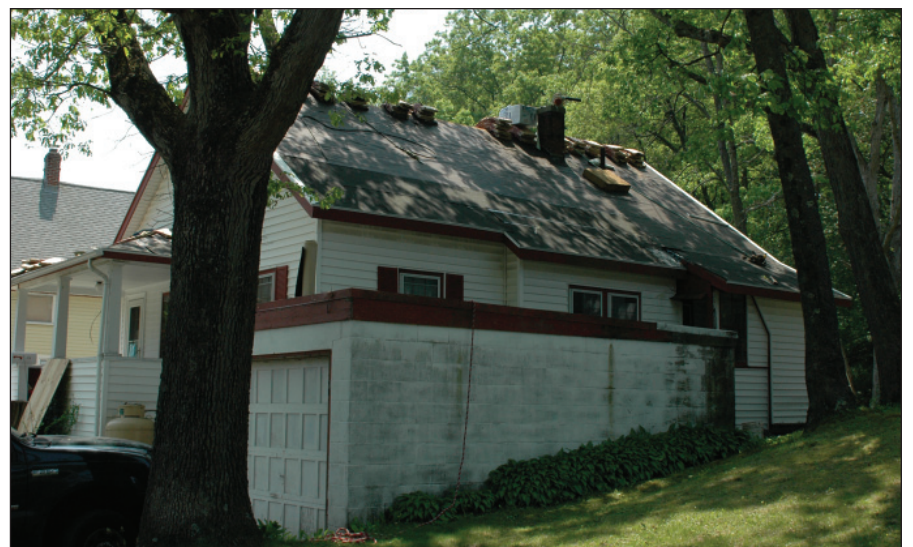
Sgt. Kelly's house during the repairs.
